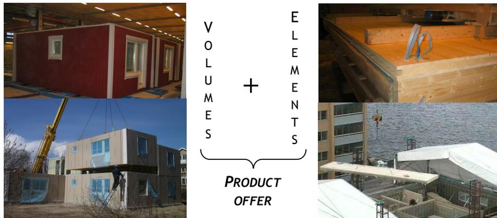
Figure 2: The *product offer* integrating prefabricated timber volumes and elements.
