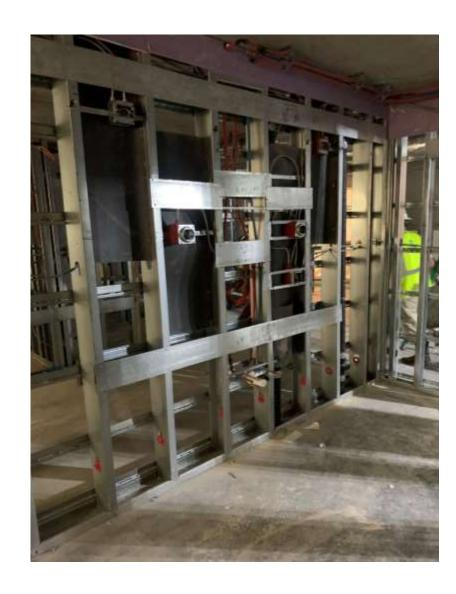
Our process and technology accommodates the penetrations for plumbing, mechanical, & electrical system components.
