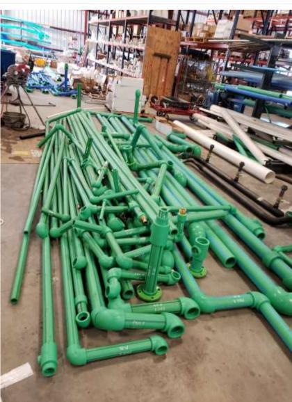
Making as many joints as possible offsite helps reduce time for installation onsite.
