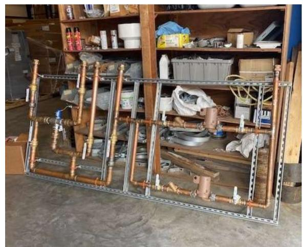
Wall mount racks for the domestic water mixing valves & recirculation pumps help reduce number of components to keep up with on-site.
